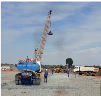
Delmas Waste water treatment works 2022 to 2023 R6.4M
